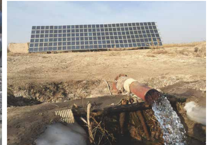
18.5kW solar pumping system in China
