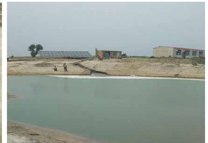
7.5kW solar pumping system in Jilin China
