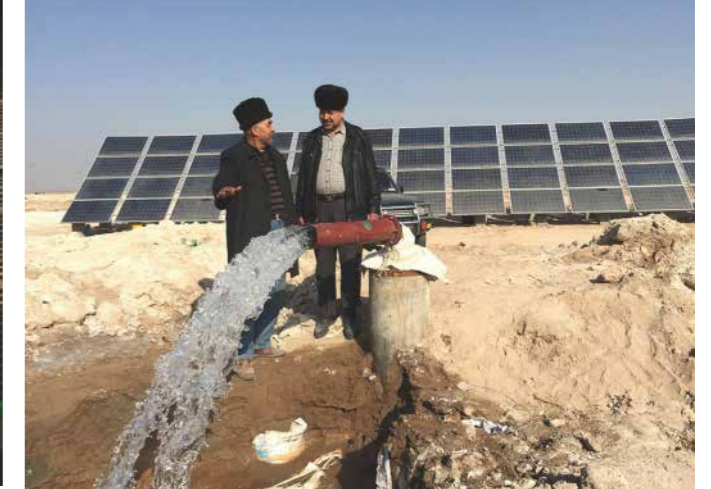
18.5kW solar pumping system in China
